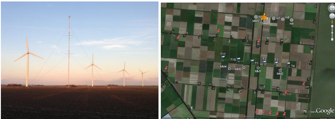
Photo of the wind turbines and met-mast (left) and Google Earth map including turbines, met-masts and in orange indication of WindScanner pattern at the ECN field site.
